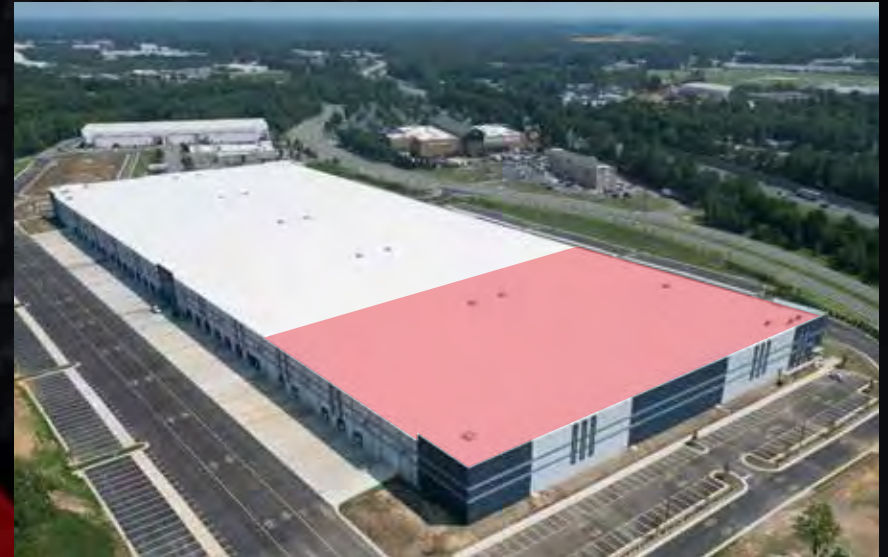
As-built Office Suite
